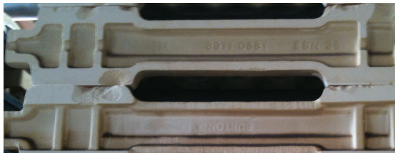
Spalling at H-cassettes
