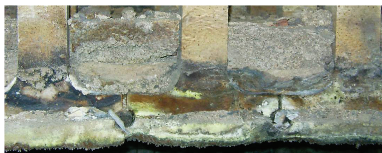
Corroded suspended ceiling due to alkali attacks
