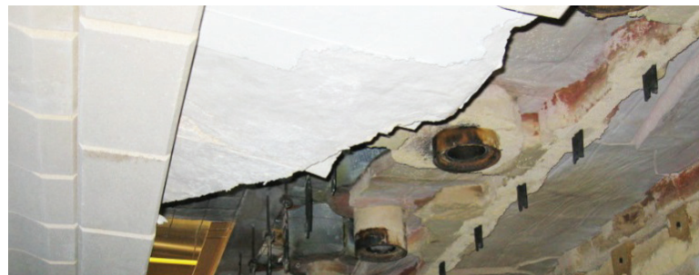
Section of suspended ceiling system dropped due to constraints
