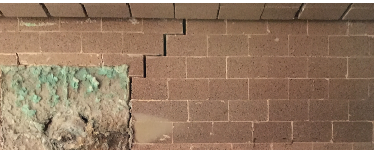
Corroded wall with step cracks
