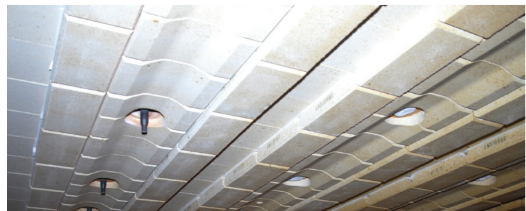
Suspended ceiling system
