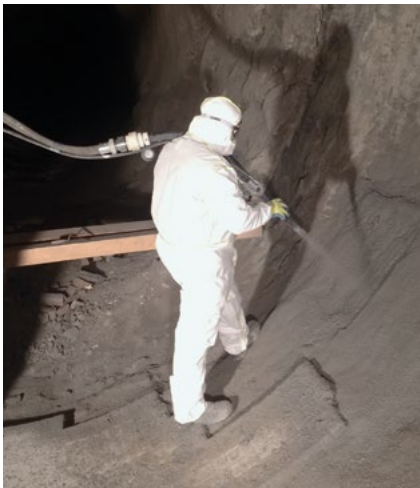
Figure 1/2: Insights into practice: Veneering of a hot spot (Fig. 1) and a protective layer in full circumference (Fig. 2), both kilns with a diameter > 5.00 m.
